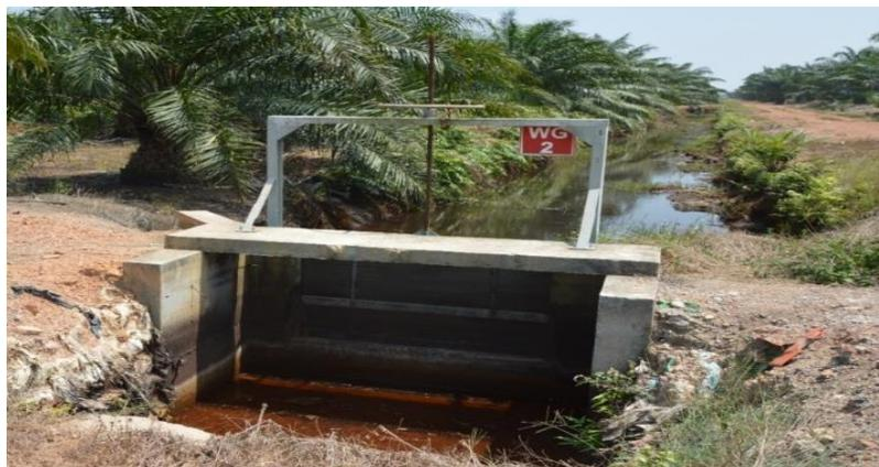
Figure 1. Installed Weir within the Peatland to Control Water Level.
